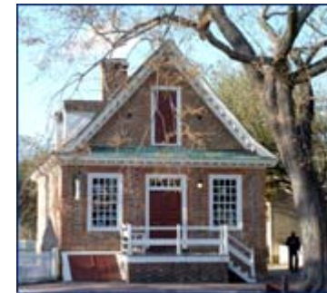
Prentiss Store (1740) 213 East Duke of Gloucester Street
